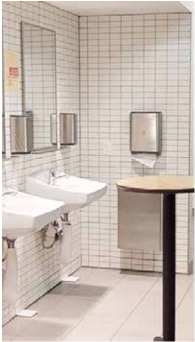
Stacked bond wall tile in the existing restrooms Photo from the Matterport virtual tour
